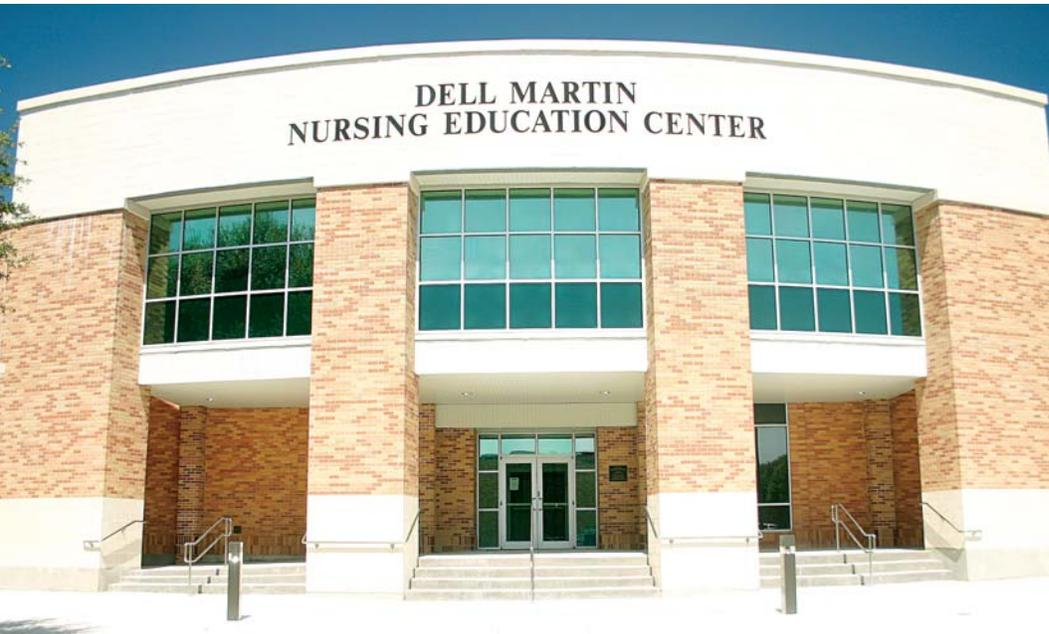
Johnson Controls subcontracted the window energy-efficiency improvement responsibility to SolArm, Inc., a LLumar dealer and a highly-qualified specialist in energy-control window film technology. Using a Department of Energy building simulation model, DOE-2, an analysis led to the selection of LLumar E-1220 low-emissivity, or low-e, window film.
